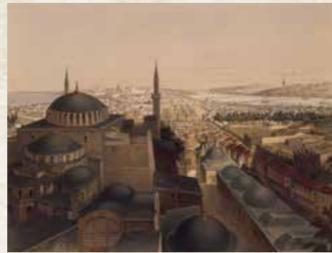
View from the upper balcony of the northeastern minaret to the West. To the right of Hagia Sophia the Keratios Bay with the bridges and in the background the Galata Tower with the Sea of Marmara on the left. On the right of the image, in the foreground, the palace of the sultan, bounded by a wall.
